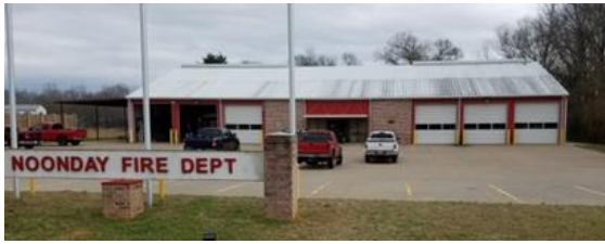
Figure 129: Noonday VFD, Station 1
